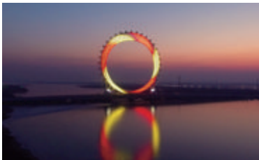
Ferris wheel Rotating Control System
