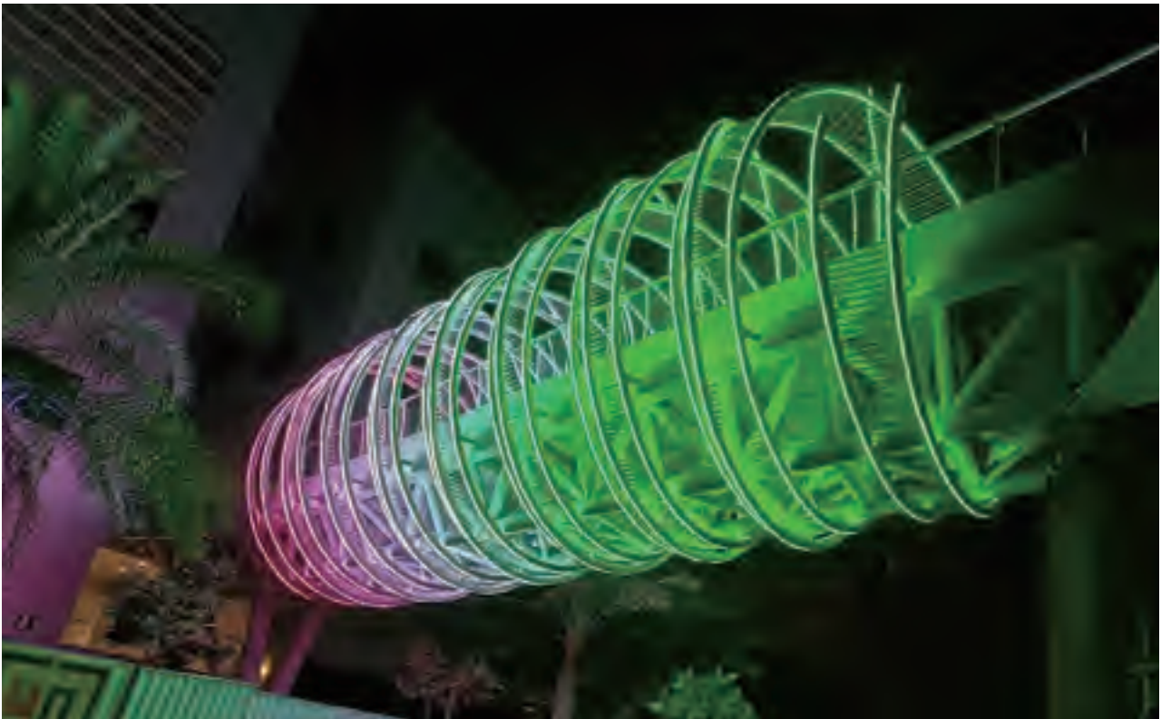
Footbridge, Abu Dhabi, UAE
